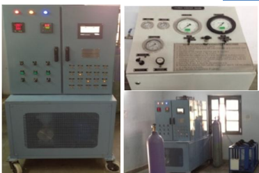
HALON Recovery, Reclamation, Recycling & Refilling Facility
