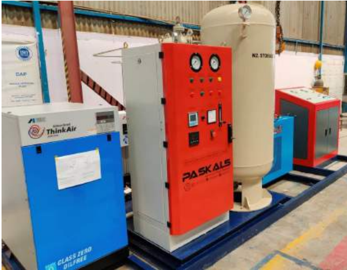
Nitrogen Generation Plant, 99.5% purity, Membrane type, Max Working Pressure 350 bar
